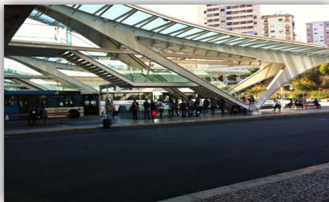
Figure 6. Transport terminal in Lisbon – a joined point of railroad, bus, metro and taxi system – platform for arrivals and departure. (Source: author, Lisbon, March 2012).
