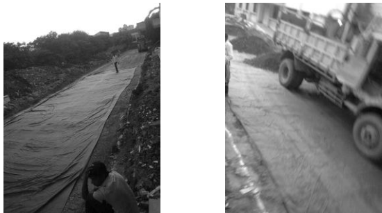
a) Geotextile above Murrum, b) GSB spreading on Geotextile
