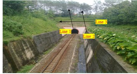
Figure 6. Dwi Bhakti Karya Railway Tunnel
